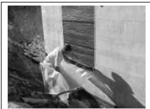
adhesive primer applied before the membrane, (3) the use of a fillet material in the inside corners, and (4) the use of a mastic to seal the edges to the footing/foundation. Failure to use these associated products with the membrane will likely cause the job to fail. Many primers and mastics will dissolve the EPS foam, so selection of one that is certified for use
