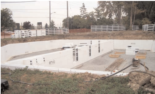
Below – school during construction.
