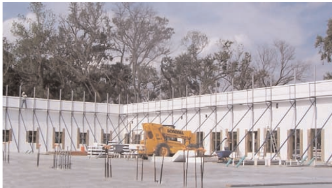
Above – Project during construction.
